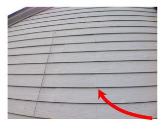
**Walls/Siding/Trim** - Caulked joints of siding are beginning to crack.
