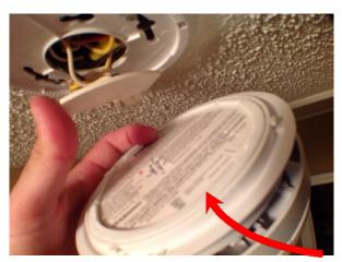
Smoke Alarm - Wrong connection for alarm, but still works.
