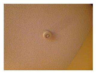
Smoke Alarm - Out of date and failed to test properly.
