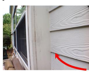
**Walls/Siding/Trim** - Caulk is separating in rear window bump out.
