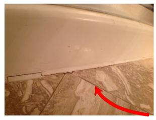
**Shower/Fixture** - Cracking Caulk on exterior of shower tray.
