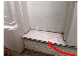
Front Door Exterior - Slight cracking of trim caulk and paint.
