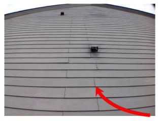
**Walls/Siding/Trim** - Caulked joints of siding are cracking.
