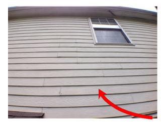
Walls/Siding/Trim - Caulked joints of the siding are cracking.
