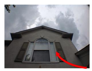
Walls/Siding/Trim - Cracking trim above window.
